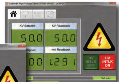
Main Control Screen
